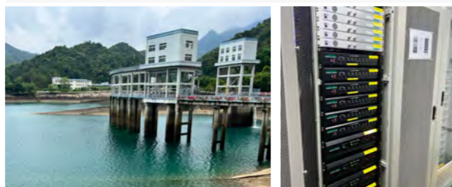
Network PA System in China Southern Power Grid
