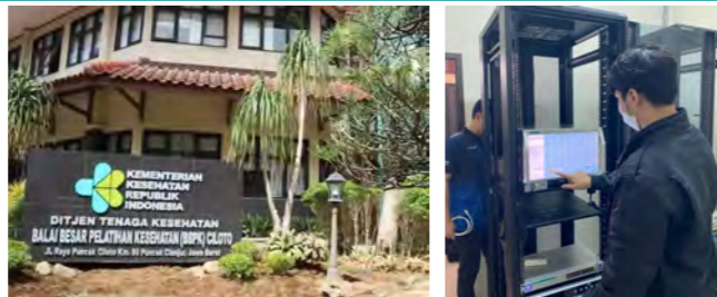
Network PA System for BBPK Ciloto in Indonesia
